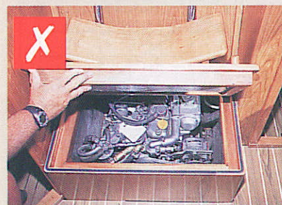
The sunken engine makes it difficult to get to the service points
