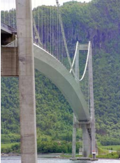
Kvisti Bridge, Norway. 9,080 m 2 . Penguard Tie Coat, Jotamastic 87 and Hardtop HB
