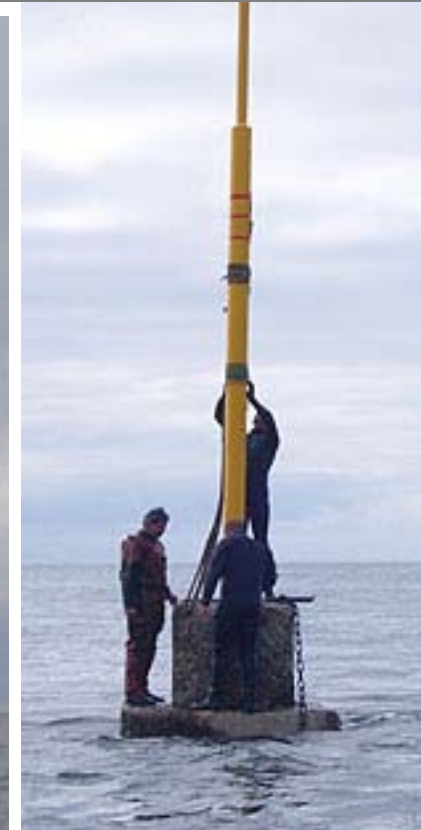
Assistance Phares & Balises : pose de la balise renforcée du "Trehu" à Groix : diam 160 - 1,6 tonne. Assistance to the Lighthouses department, in very shallow waters.
